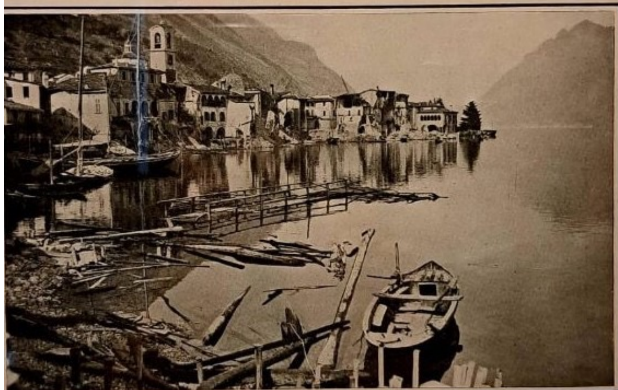
VIEW OF TAVERNOLA AFTER THE HURRICANE The little town of Tavernola, about 14 miles from Florence on Lake Isèo, was recently visited by a disastrous hurricane, resulting in a scene of positive devastation
